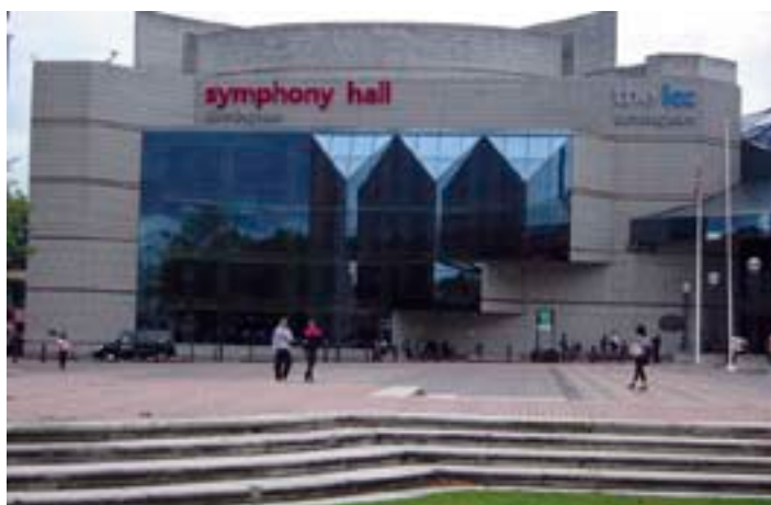
The forecourt of the International Convention Centre.
